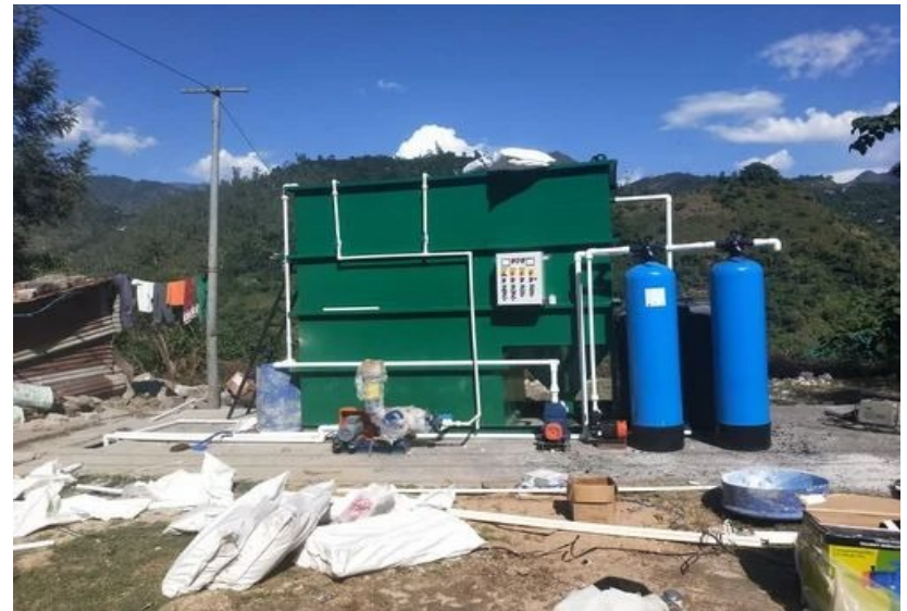
SEWAGE CUM EFFLUENT TREATMENT PLANT
